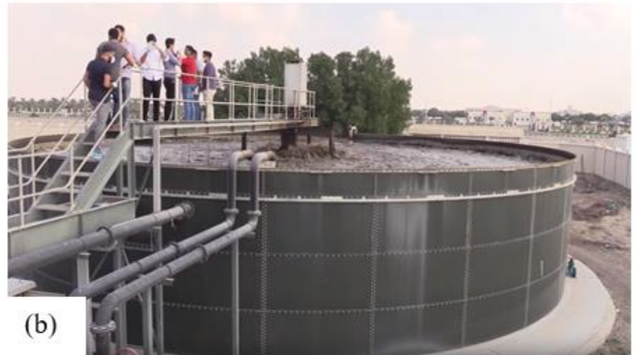
(a) University City Wastewater Treatment Plant layout, and (b) primary clarifier of the treatment plant
