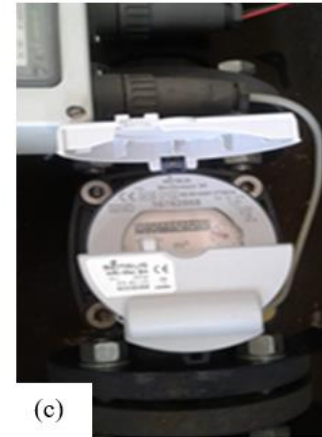
Figure 2: (a & b) Faucet aerators: Automatic & low flow nozzle faucets installed in all academic buildings including on-campus mosques and (c) Smart water meter to manage water usage
