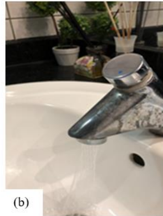
Figure 2: (a & b) Faucet aerators: Automatic & low flow nozzle faucets installed in all academic buildings including on-campus mosques and (c) Smart water meter to manage water usage
