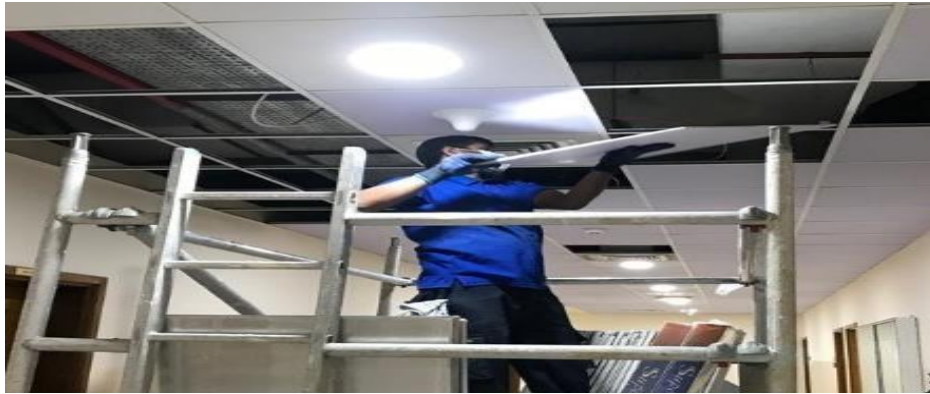
Figure 20: Replace light bulbs with led panels.
