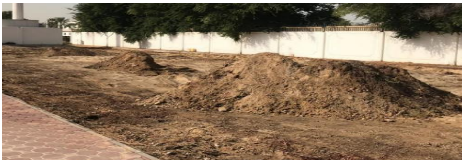
Figure 54: Sand provided by Sharjah Municipality.
