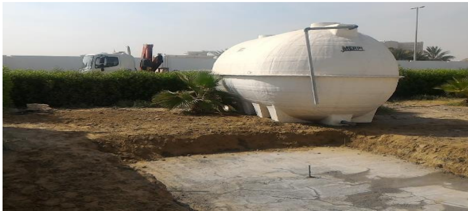
Figure 50: Water tank in the greenhouse.
